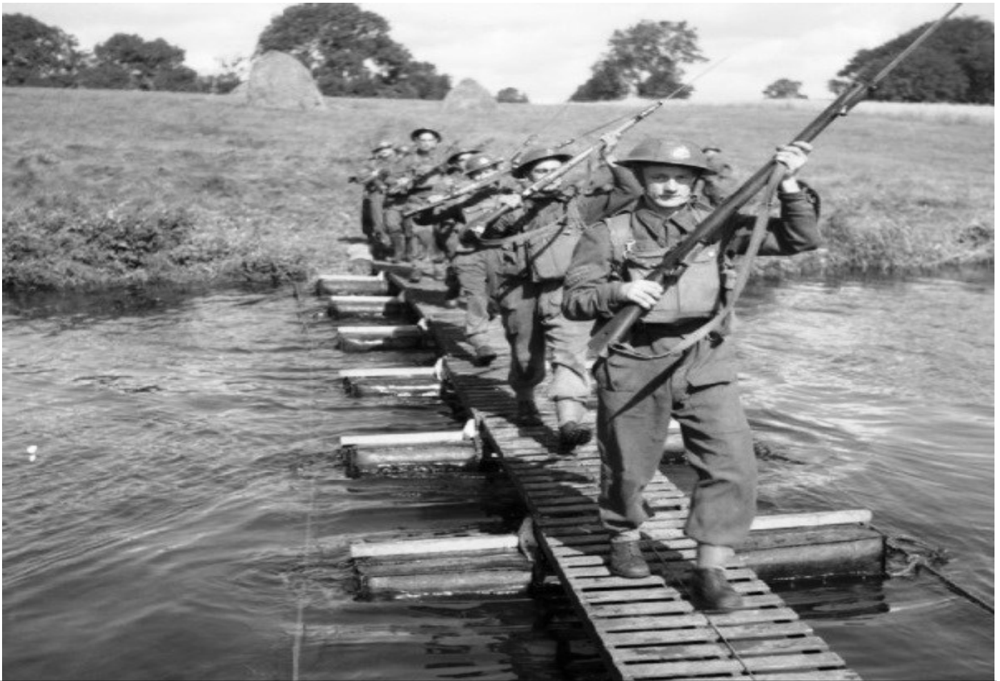
Soldiers crossing a river using a kapok footbridge. Kapok was a light cotton-like substance that remained afloat even when punctured with rifle fire.
