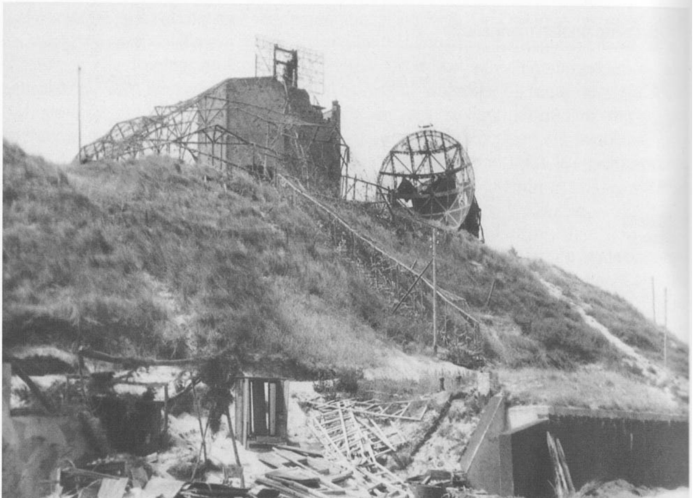
Above: Radar post Monika to the south of Westkapelle. On the left is 'Calais' (Fu.M.O.2), to the right is Wurzburg radar 'Riese' (Fu.M.O.214 (Seetakt)). Only the radar antenna of 'Calais' is visible, the rest of the radar apparatus is behind the large wall to protect it from bomb and grenade shrapnel.
